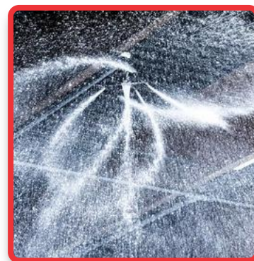
One Seven Stored Energy System
