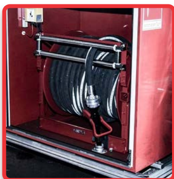
One Seven Wall Hydrant
